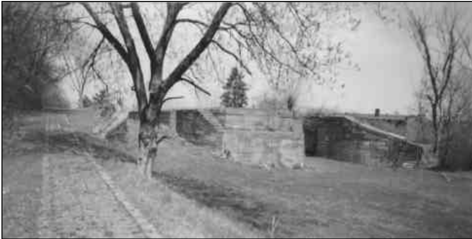
Massive stone structures of Lock 17
