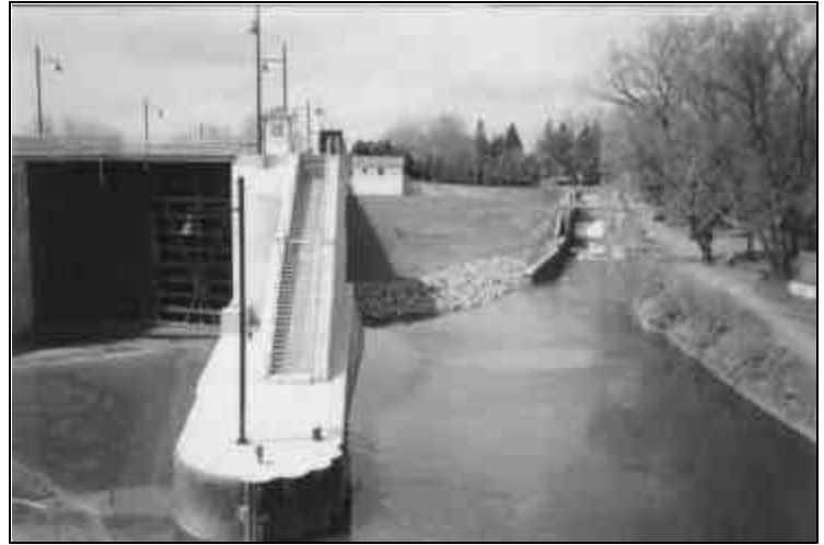
Erie Barge Canal Lock No. 2 and Cross-Cut Canal
